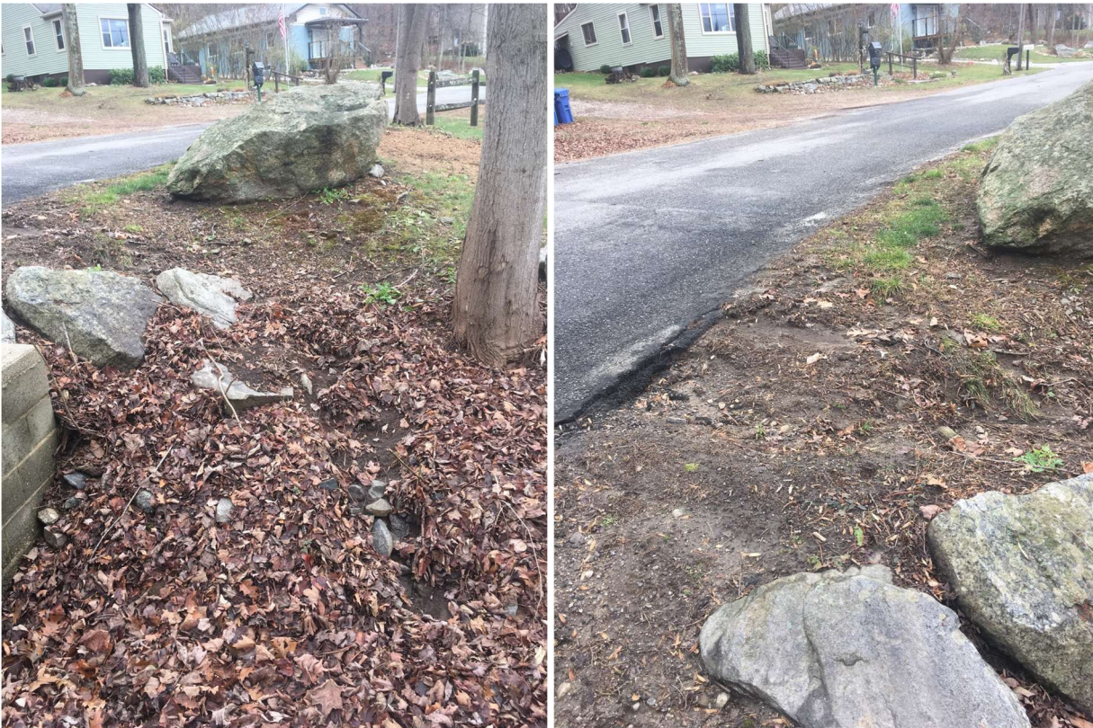
Pictures of erosion near L32, Address Deepwood 12, 15 Lebanon
