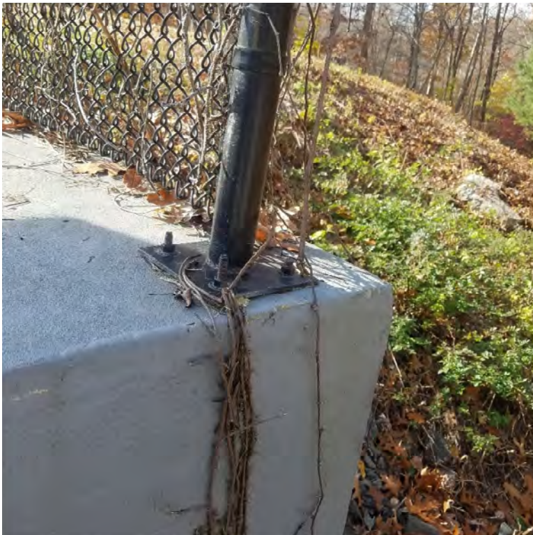
Photo 21j – For comparison purposes, the end post atop the left side wing wall has a bracket attachment rather than being set into the wall. No concrete issues are present.
