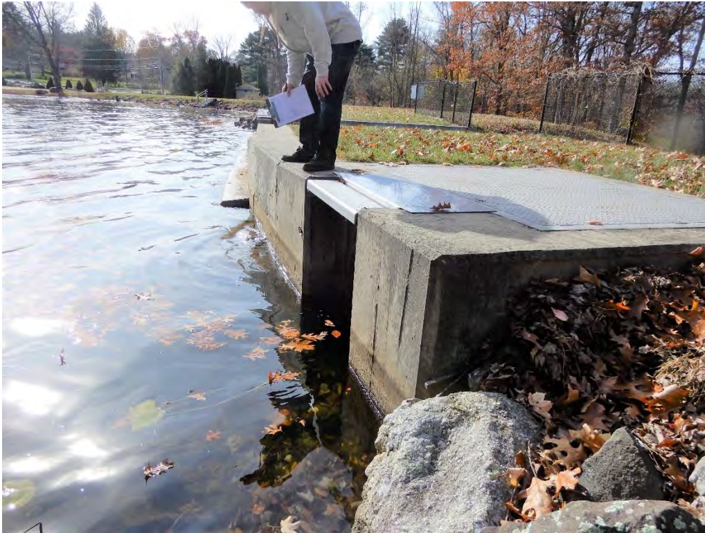
Photo 16a & 19a – The upstream face of the intake structure.
