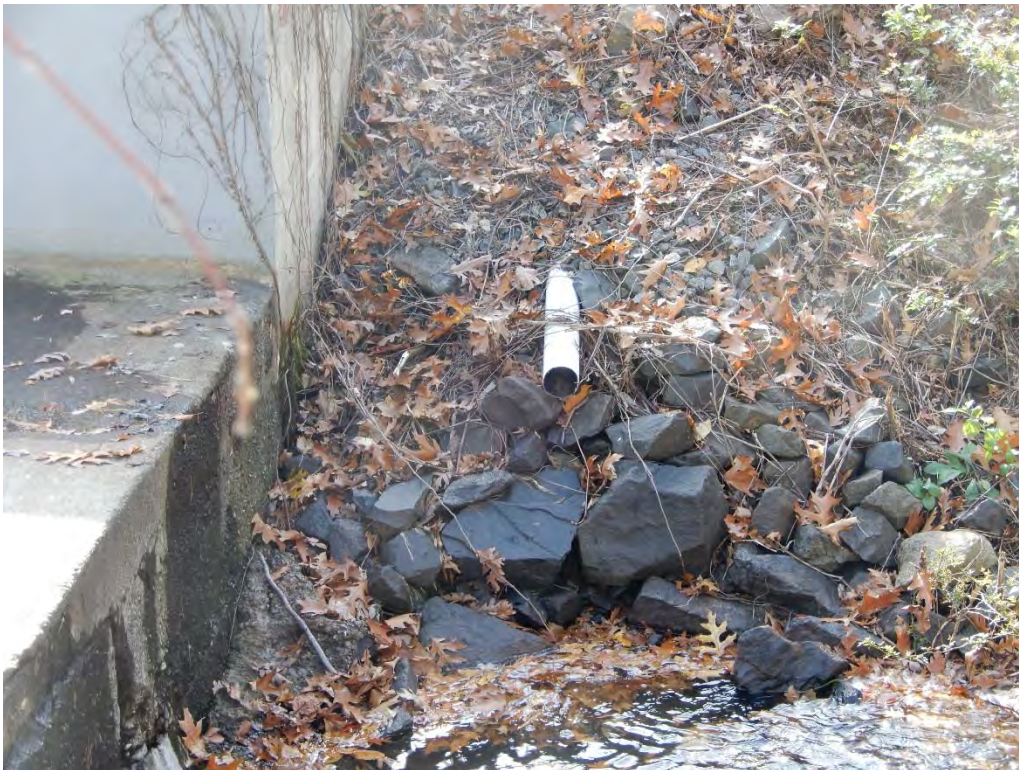
Photo 19d – The downstream outlet end of the left side toe drain pipe, discharging into the stilling basin at the downstream base of the spillway.
