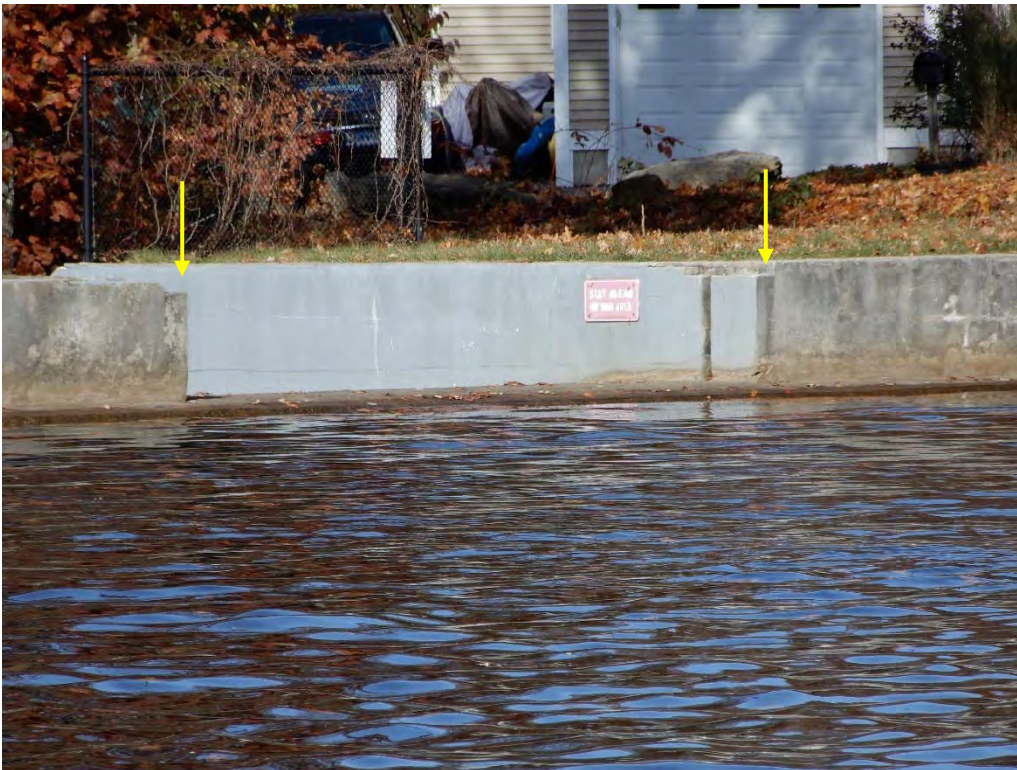
Photo 9a – The spillway approach as seen from the upstream side. The two arrows point to the upstream training wall corners.
