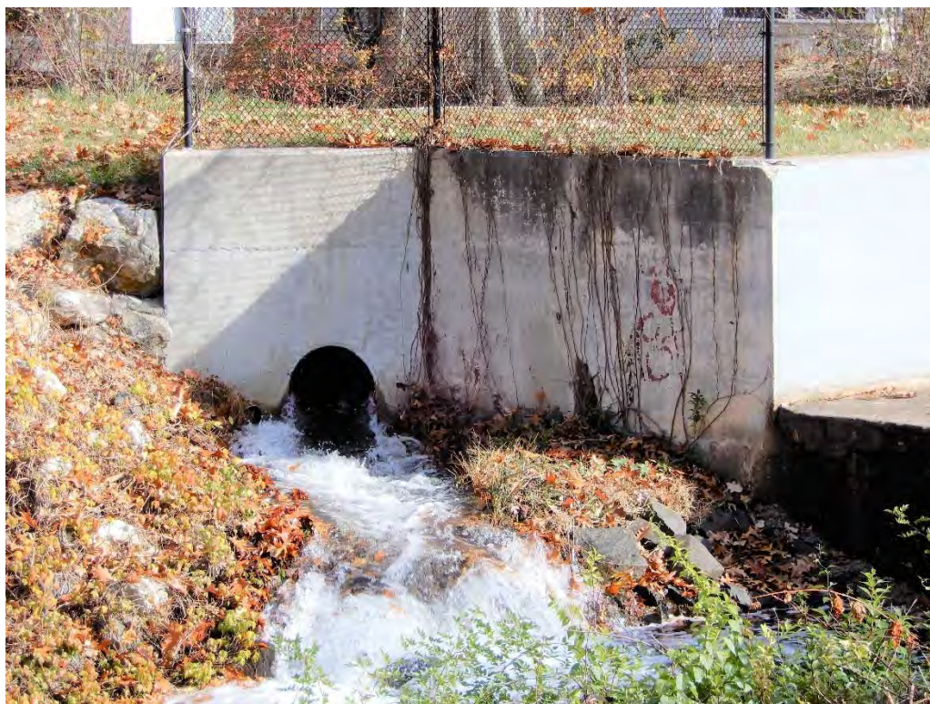
Photo 19b – An overview of the downstream face of the right side wing wall, with the low level outlet pipe situated near its base.
