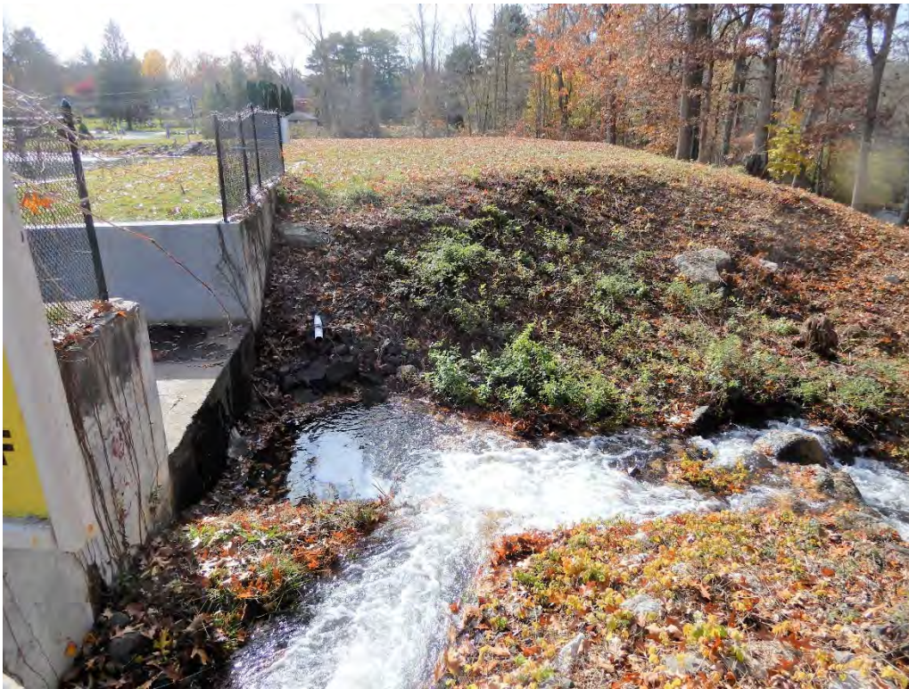
Photo 14 – The stilling basin at the downstream end of the spillway discharge chute. The area is composed of small riprap stones and natural channel base materials, and is generally stable.
