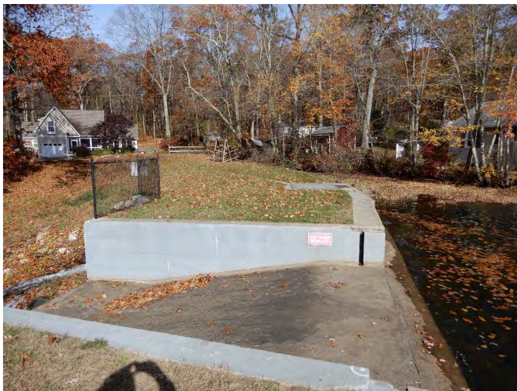
Photo 11 – The right side spillway training wall.
