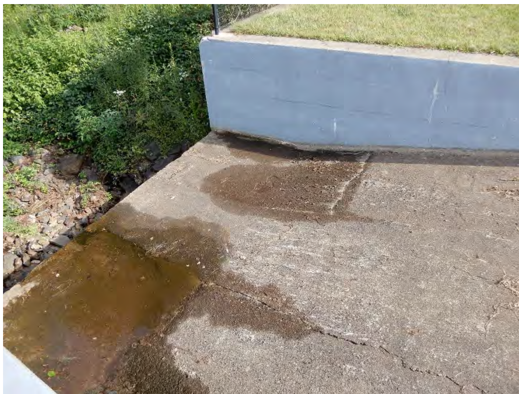
Photo 21b – A closeup view of seepage collecting at the base of the spillway chute.
