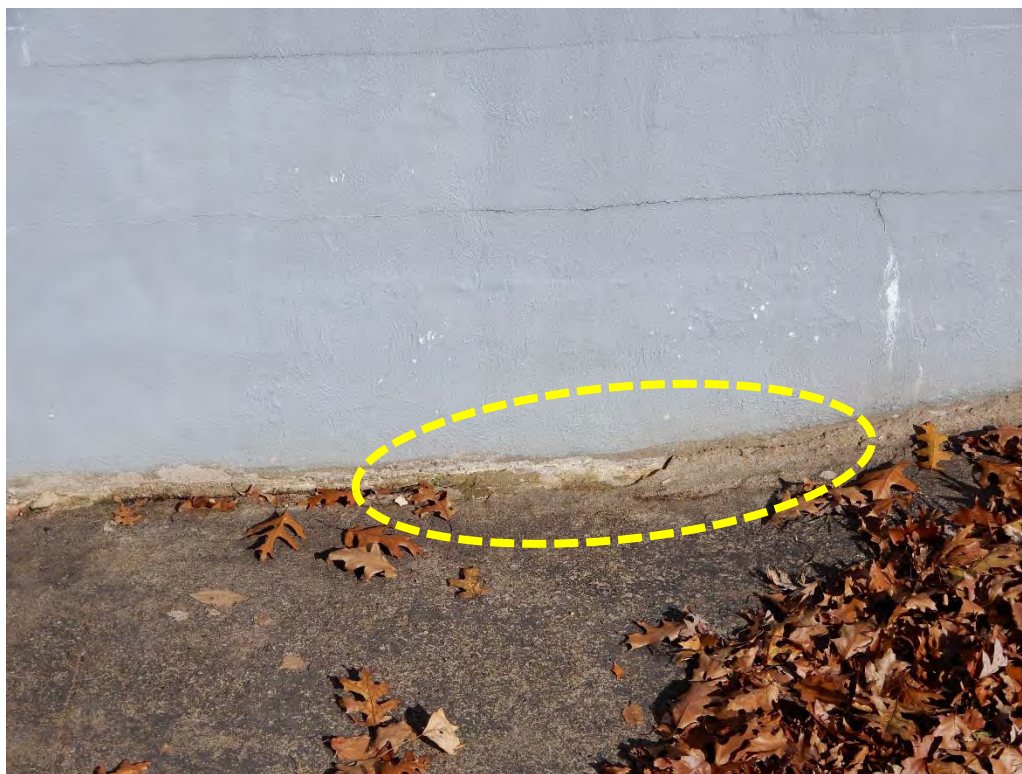
Photo 21o – A small area of cracked grout at the joint along the base of the right side training wall near the bottom of the apron.
