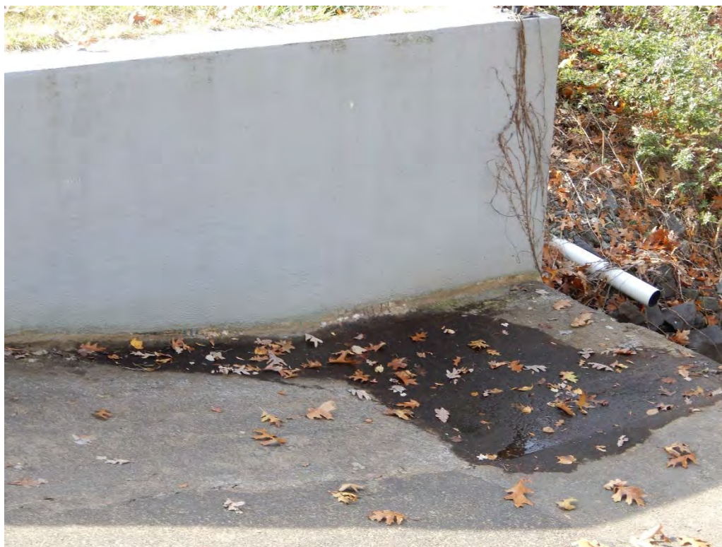
Photo 21c – Another view of the seepage at the base of the left side of the apron.
