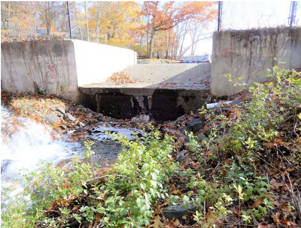
Photo 10 – An overview of the spillway from the downstream side. Flow on the left is being discharged from the low level outlet.
