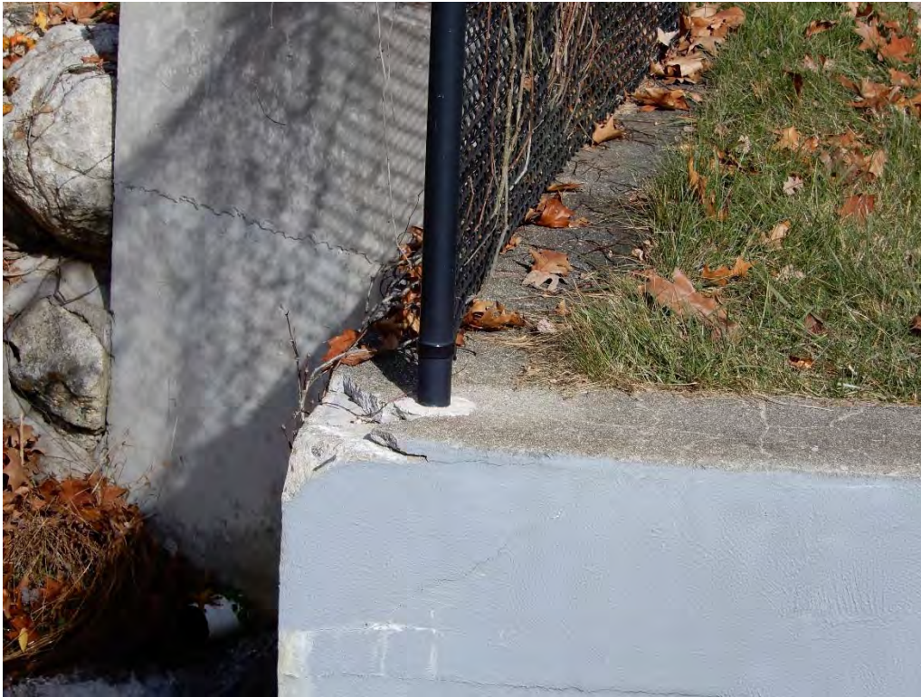
Photo 21i – Cracking and deterioration at the downstream corner of the right side training wall. This issue appears to have been caused by the adjacent fence post set into the concrete with expansive grout, which has prompted the cracking and chipping.
