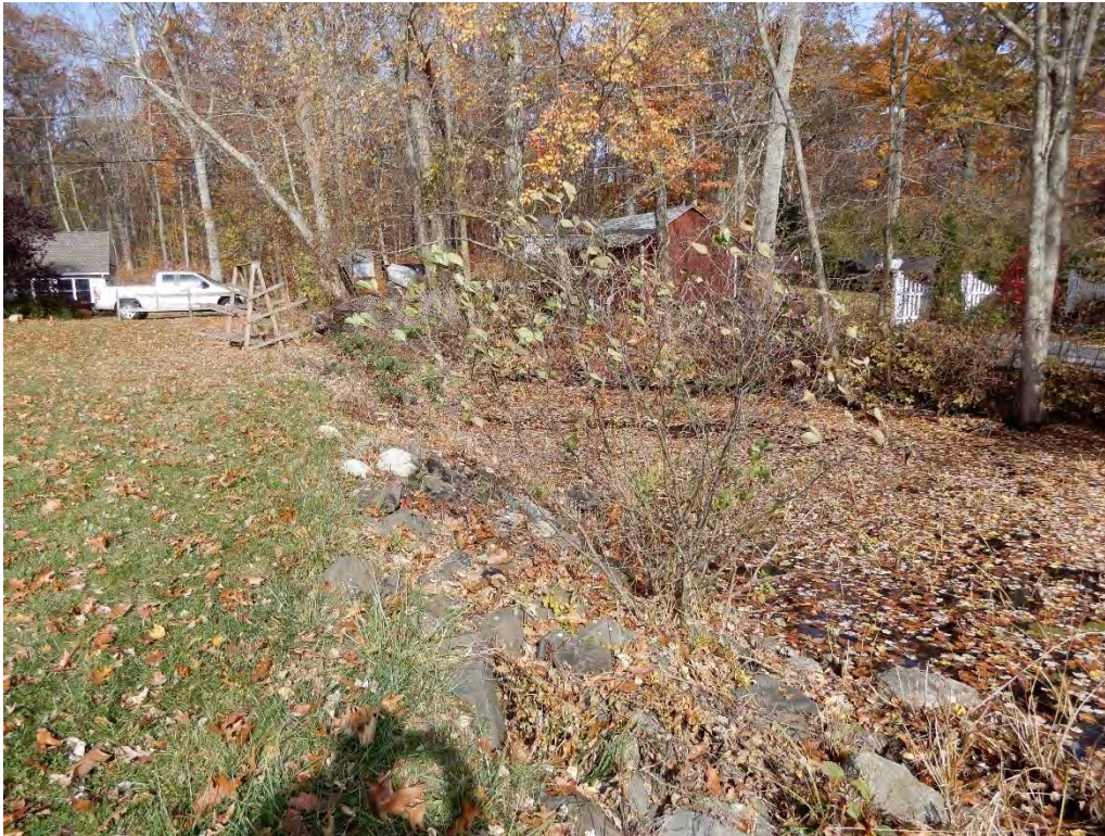
Photo 3c – A few of the right upstream embankment as seen from the right side of the spillway. Brush, such as that shown in the foreground, should be removed from the embankment
