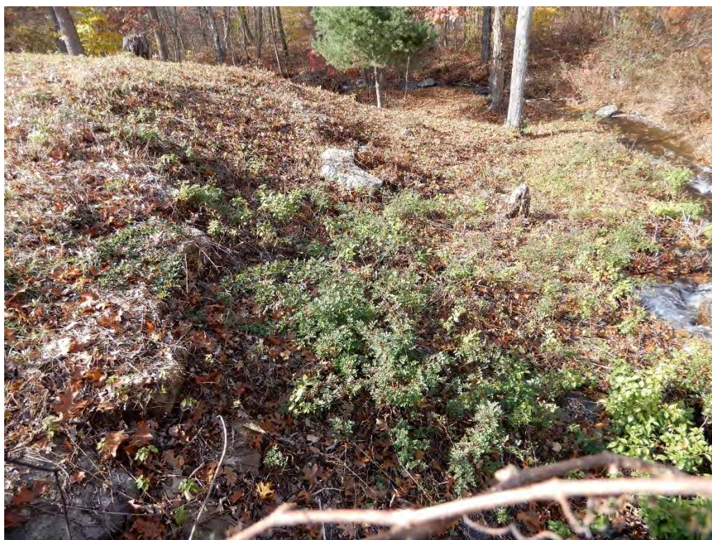
Photo 21d – Shrubby along the downstream embankment face left of the spillway. Although minor in scope, this area should be cleared, and a grass cover reestablished in line with other embankment areas for ease of maintenance.
