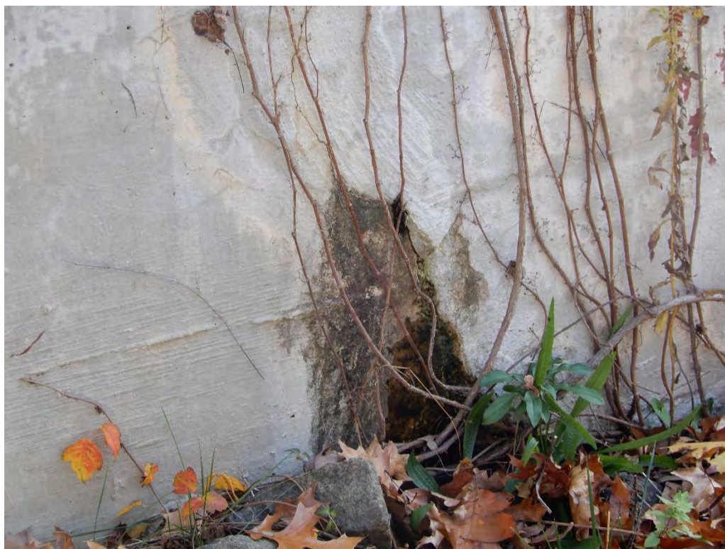
Photo 21k – A section of minor concrete deterioration along the downstream face of the right side wing wall. This area should be cleared and patched.
