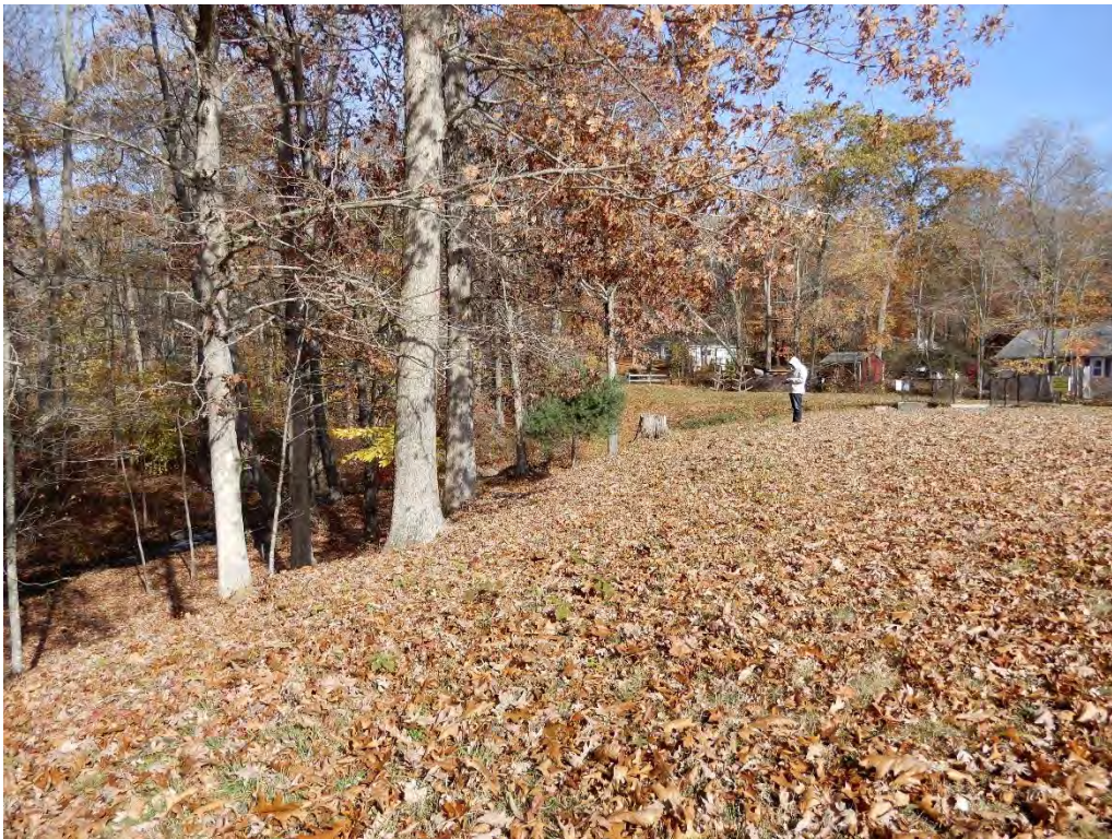
Photo 21f – Trees present along the left downstream embankment face. This growth should be cleared from the embankments and areas with 25' thereof, and a grass cover established and maintained.
