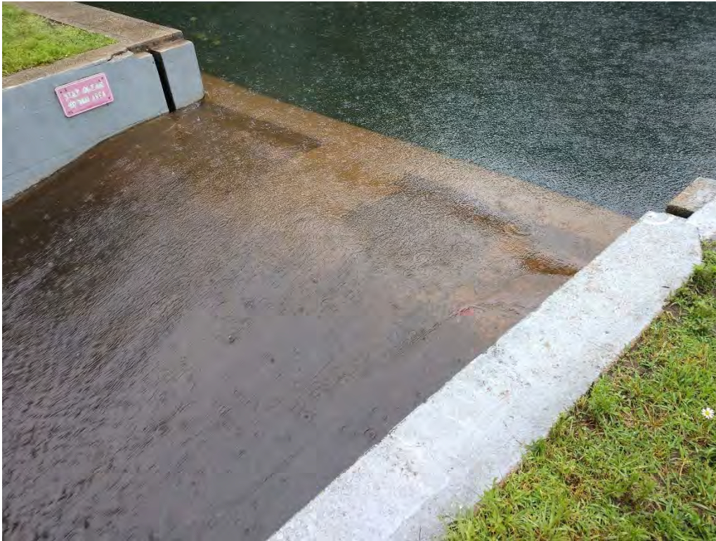
Photo 13 – Looking down at the spillway weir, under light flow conditions.
