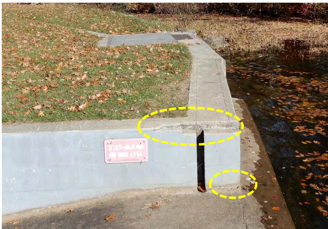
Photo 21l – Two concrete areas with minor issues, one a longitudinal crack at the top and a small open crack at the right bottom base.
