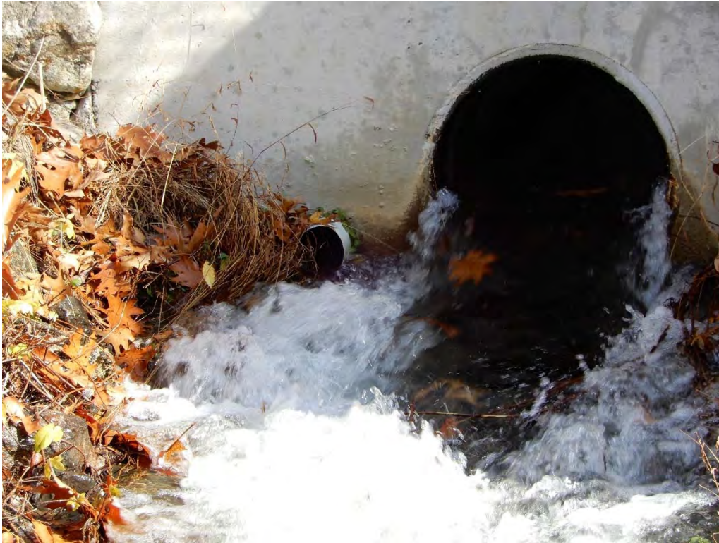
Photo 19c – A head on view of the downstream ends of the low level outlet pipe and toe drain pipe.
