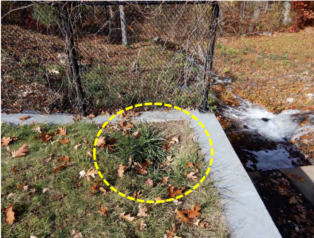
Photo 21e – A minor depression adjacent to the left side training and wing walls. This area should be filled in and monitored, particularly as it is situated above a section of the training wall wherefrom minor seepage emanation was observed.
