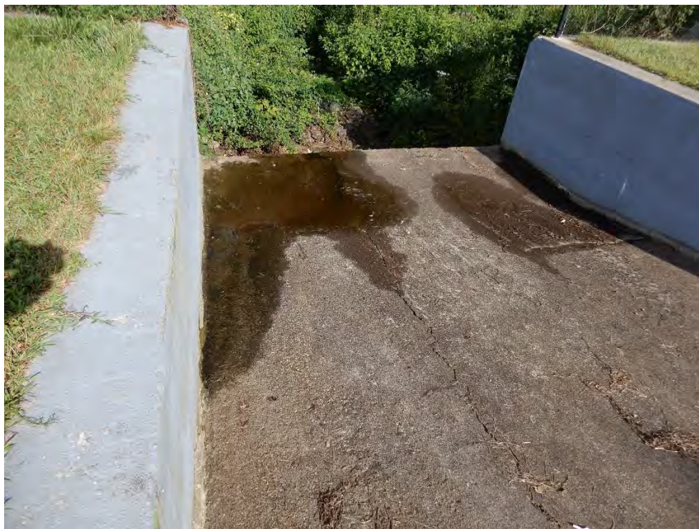
Photo 21a – An overview of the spillway discharge apron, showing seepage near its left and right side base, apparently emanating from the bottom interface with the training walls. Also note thin cracks along the line of flow toward the center of the apron.
