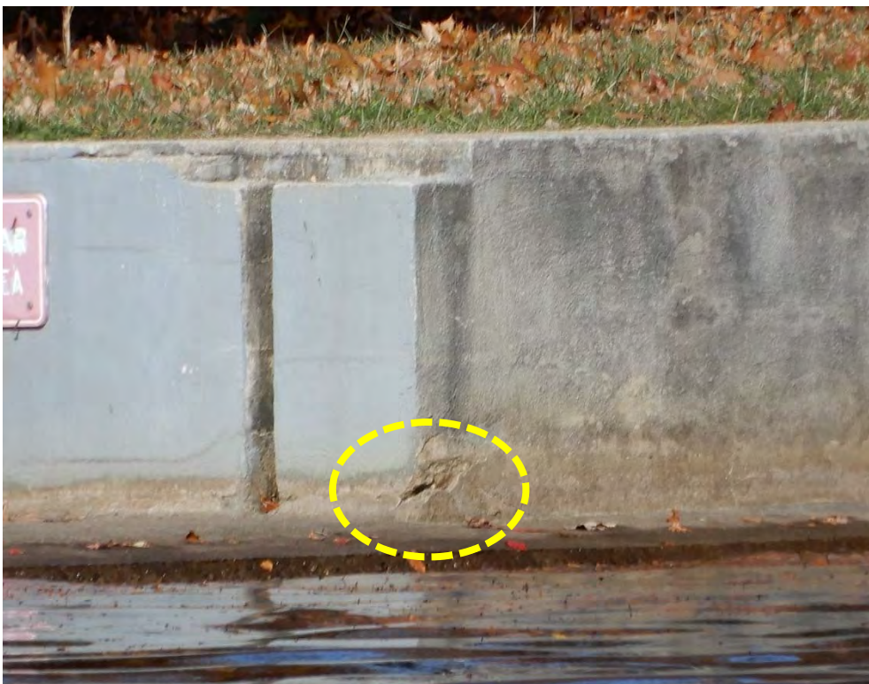
Photo 21n – A closeup of the lower right side crack issue at the base of the training wall.
