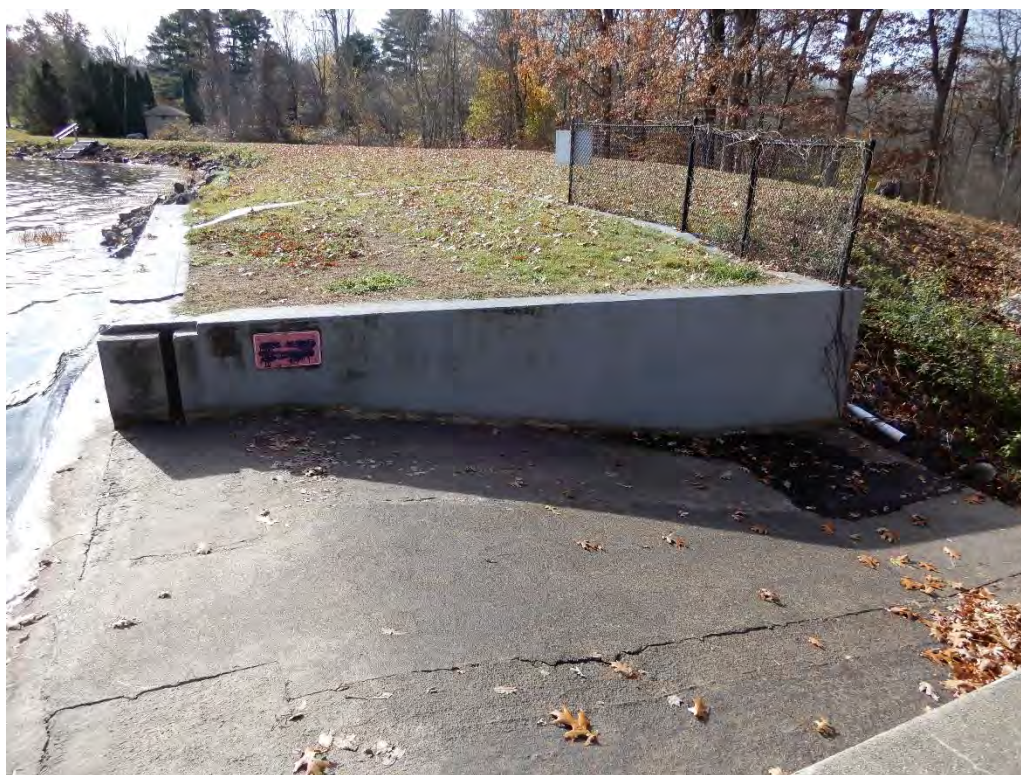
Photo 12 – The left side spillway training wall.
