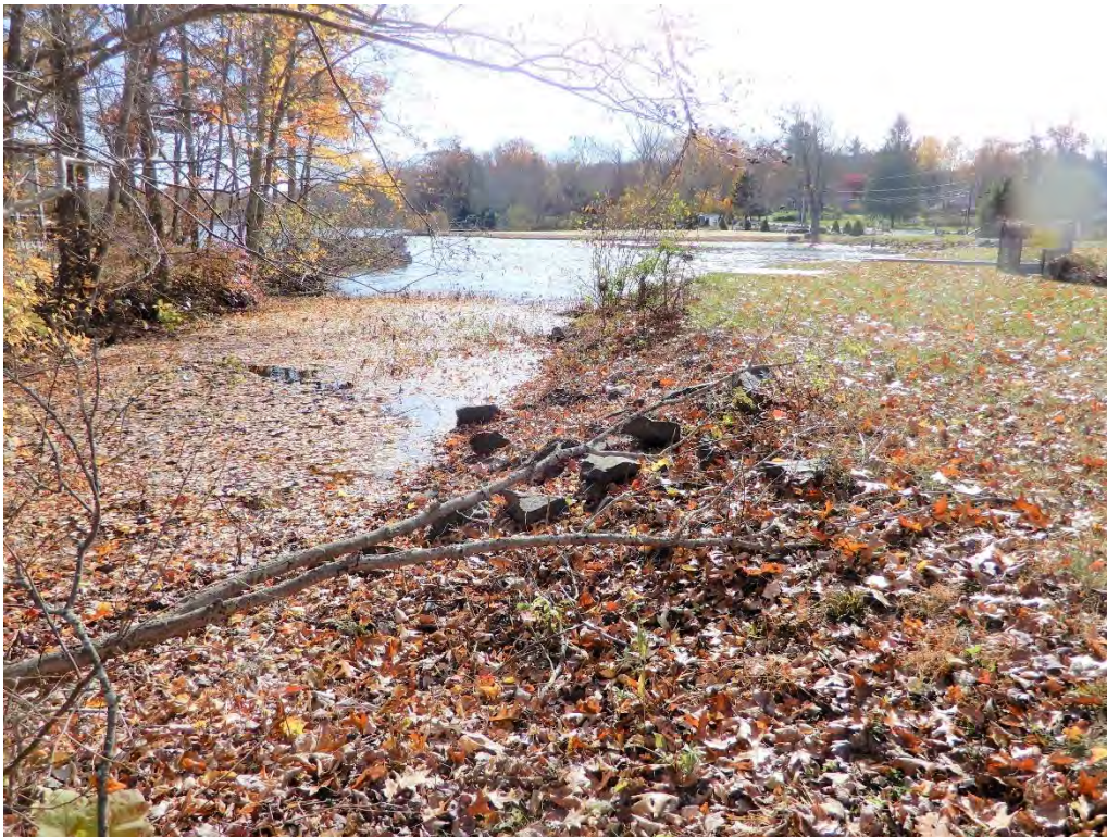
Photo 3b – The right upstream embankment. Although there is some leaf litter present from trees on the opposite shoreline, the embankment here is stable and well maintained.
